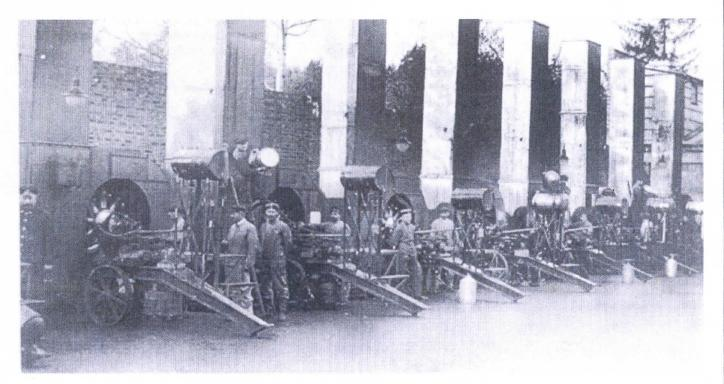
Motorenfabrik Oberursel – engine acceptance testing
